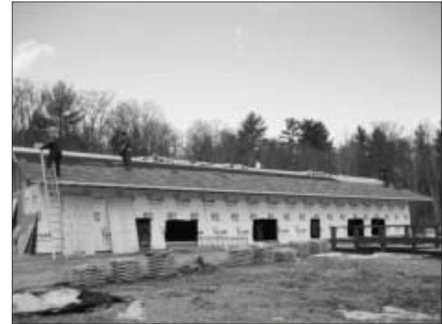
Construction at Lions Camp Dorset Winter/Spring 2008
